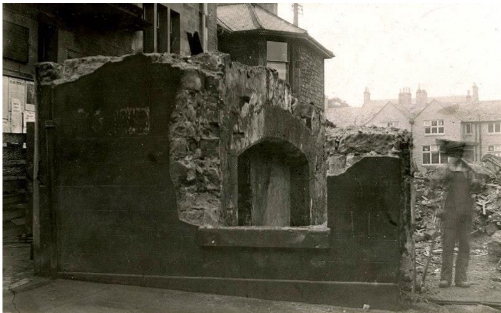
The fireplace comes into view after the majority of the demolition work was completed, and the thickness of the wall behind it also becomes evident. The area was being cleared in 1935, to make way for an entrance to the new police houses seen in the background. Copyright: The David Moore collection, Guild of Freeman, Berwick-upon-Tweed.
