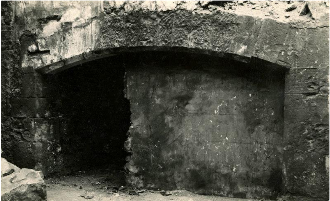
The huge size of the fireplace becomes apparent from this photograph. Also what the photograph appears to show is that the fireplace was blocked up by stone at some point, as the large gap on the left shows. Copyright: The David Moore collection, Guild of Freeman, Berwick-upon-Tweed.
